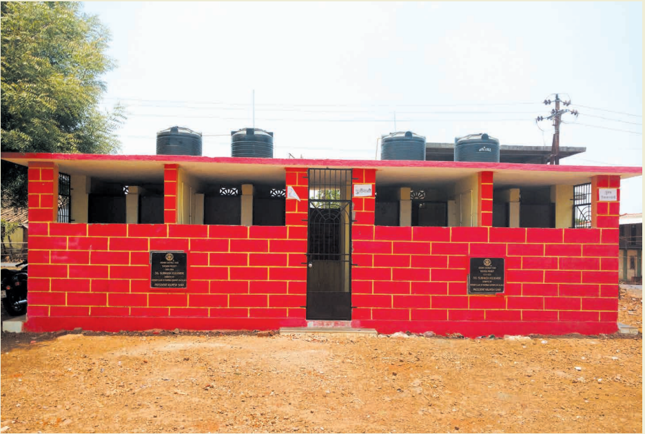
Rotary International, Sukhada Project, Thane, Maharashtra
