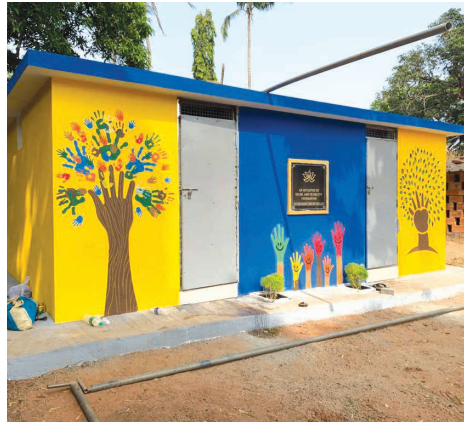
Combined school toilets blocks, Kappu, Udupi District, Karnataka. Partner - BR & CR Shetty Foundation
