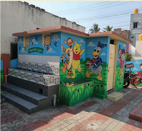
236 girls toilet blocks in Chittoor District, Andhra Pradesh, Partner- MUFG
